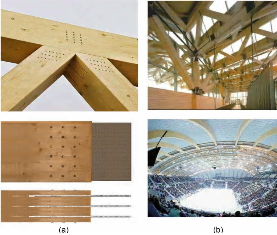
Figure 1 (a) Dowel-type joints with steel plates and steel dowels. (b) Two glulam structures in which dowel-type joints are used. The pictures are reproduced by the permission of Svenskt Limträ AB ([www.svensktlimtra.se](http://www.svensktlimtra.se)).
